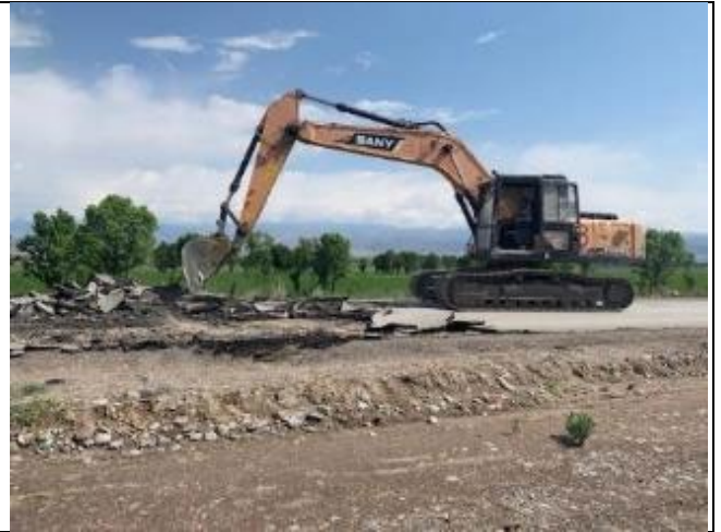
Photo 50. Scarifying of asphalt concrete pavement at km 74+550.
