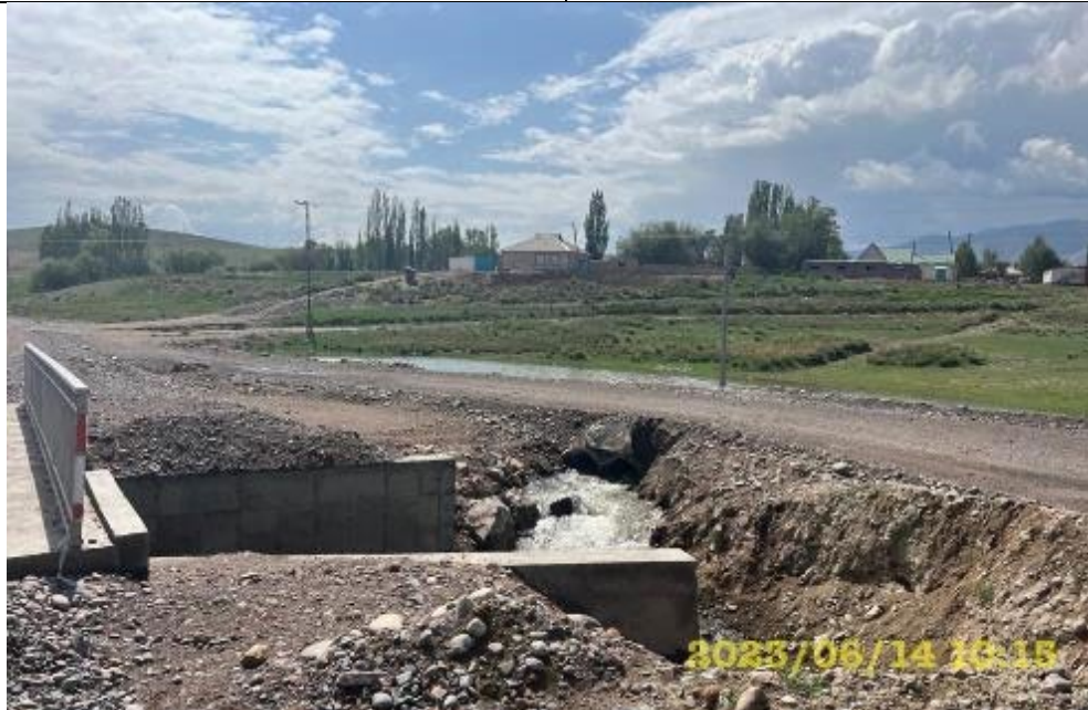
Photo 94. Lot 2. Mukandyn-Suus River bridge, km. 68+040. There are no protective measures to prevent soil from entering the river during construction works.
