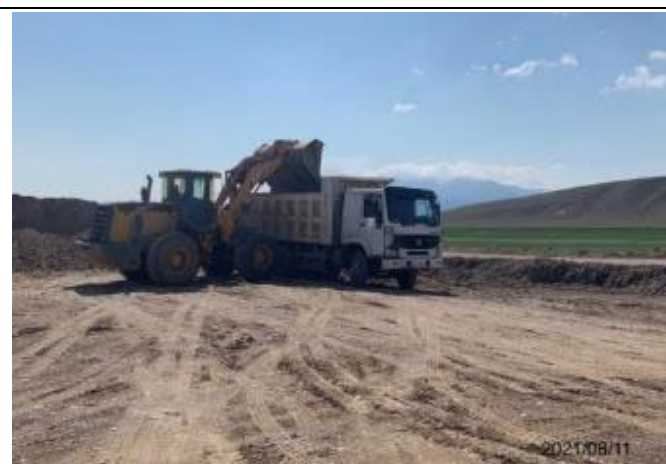
Photo 34. Quarry at km. 81+200, loading of moistened material.
