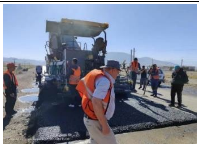
Photo 75. Lot 2. SMA arrangement km 81+675-82+000 RHS.
