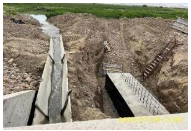
Photo 95. Lot 2. Mukandyn-Suus river bridge, km. 68+040 Water diversion is provided to prevent soil from entering the river during construction works.
