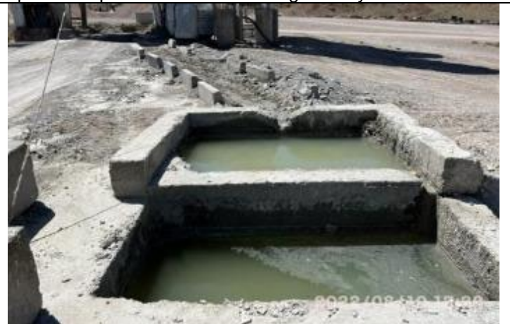
Photo 115. Lot 1. 3-chamber primary wastewater treatment tank. Concrete mixing plant.
