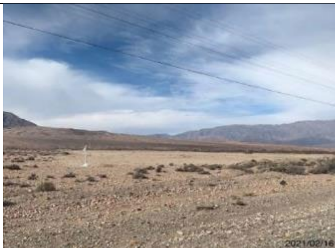
Photo 32. Lot 1. The topsoil was removed from quarry site at km.9+000, the quarry boundaries were marked by installing white posts with flags
