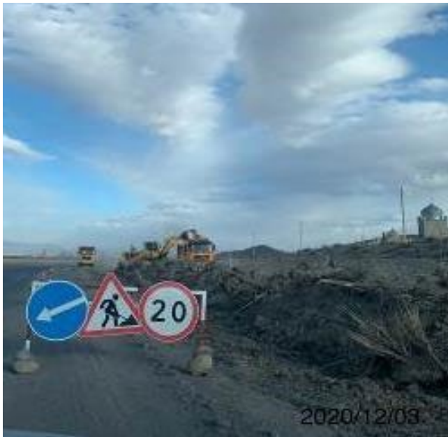
Photo 13. Lot 2. Removal of soil and vegetation layer from roadside on section km. 83+600 - km. 85+000.
