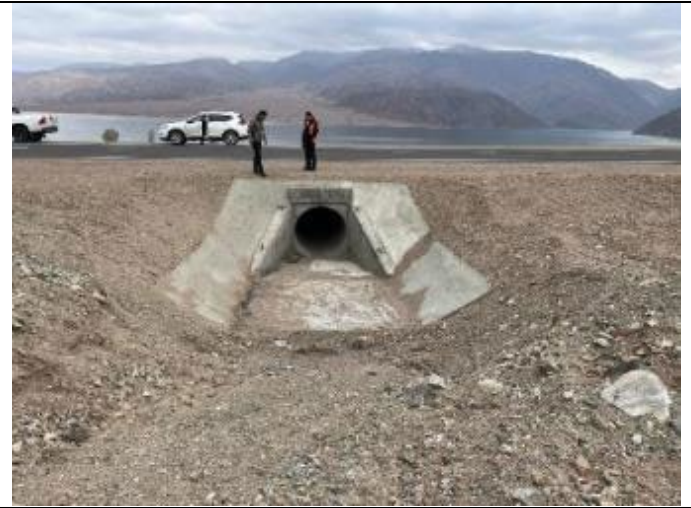
Photo 104. Lot 1: Culvert cleaning, km 33+869.
