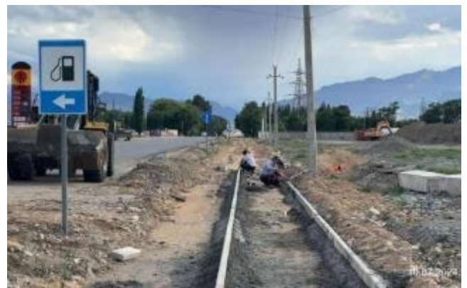
Photo 2. Installation of curbs for sidewalk at km 1+360-1+800 RHS. July 2024.
