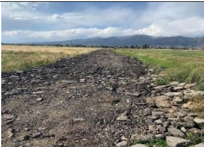
Photo 58, 59. Improvement of peripheral street with old asphalt (laying and leveling) in Cholpon village.
