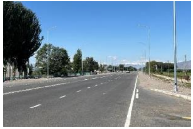
Photo 18. Completion of shoulders, curbs and lighting. August 2024
