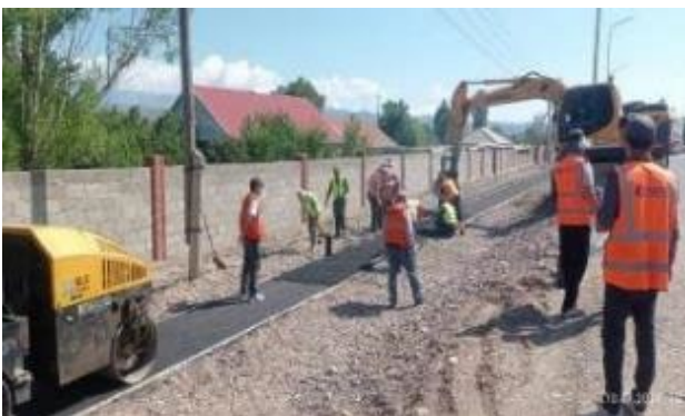
Photo 15. Arrangement of asphalt on sidewalk, km 70+100-70+740 LHS. July 2024.
