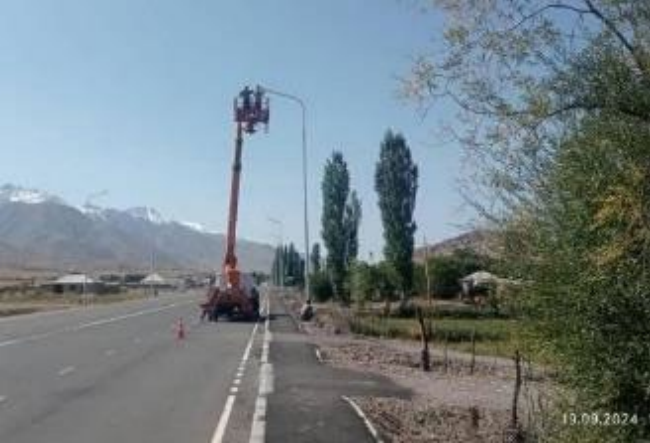
Photo 19: Installation of lighting devices at km.86+100-87+700 BS. September 2024
