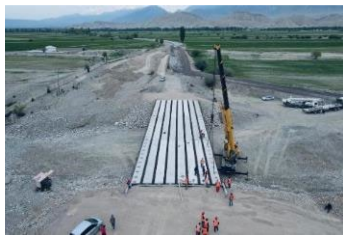
Photo 93. Lot 2. Photo 6. Construction of a bridge over the Joon-Aryk River at km. 65+410, installation of slabs.
