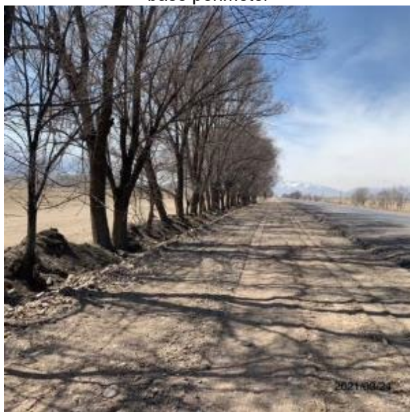
Photos 19 and 20. Road shoulders with removed soil layer
