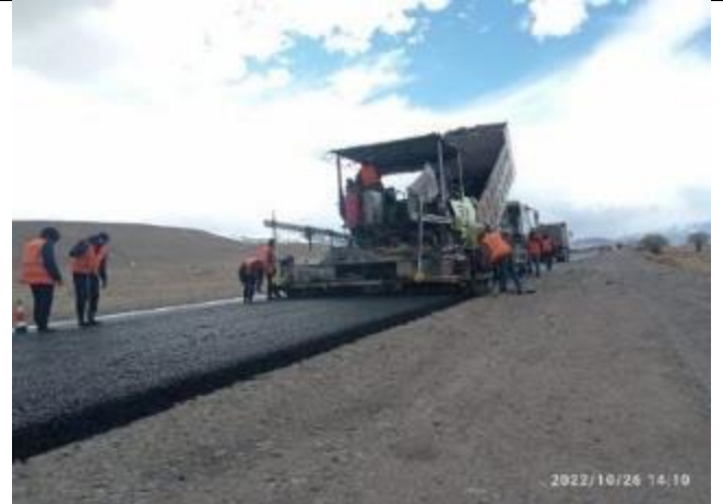
Photo 75. Lot 2. SMA arrangement km 81+675-82+000 RHS.
