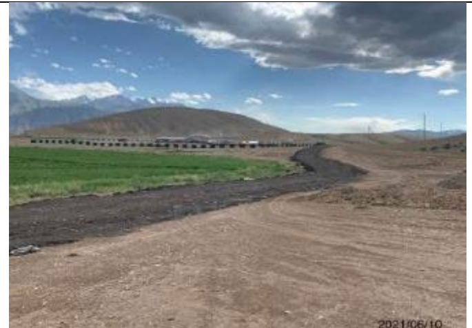
Photo 55. Lot 2. Old asphalt, to prevent dust formation, laid on the technological ground road to Crushing plant.
