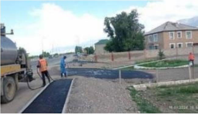
Photo 17: Application of prime coat on exits at km 65+648. July 2024
