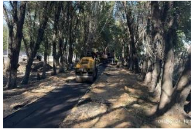
Photo 20. Asphalt paving on sidewalk, km 2+050-2+414 LHS. September 2024.
