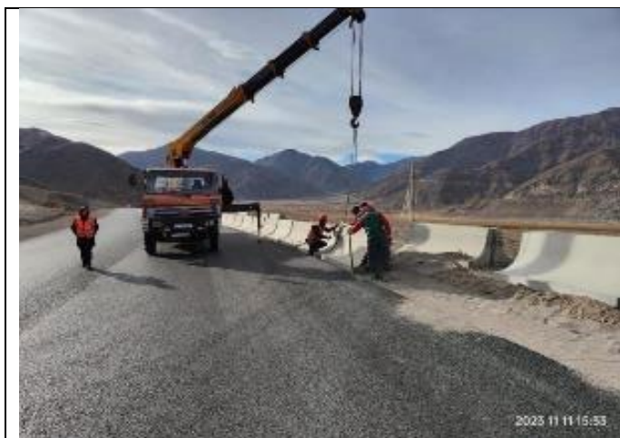
Photo 109. Installation of parapets on 40+700-40+870 RHS.
