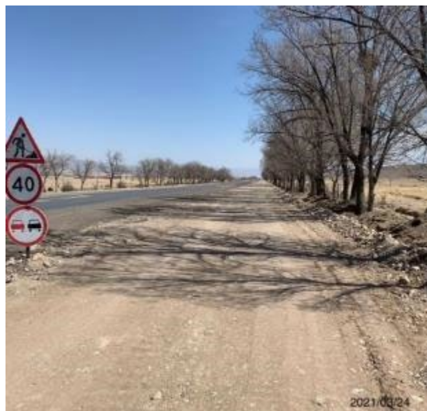
Photos 19 and 20. Road shoulders with removed soil layer
