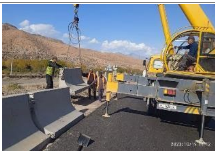
Photo 110. Installation of parapets at km.11+200.
