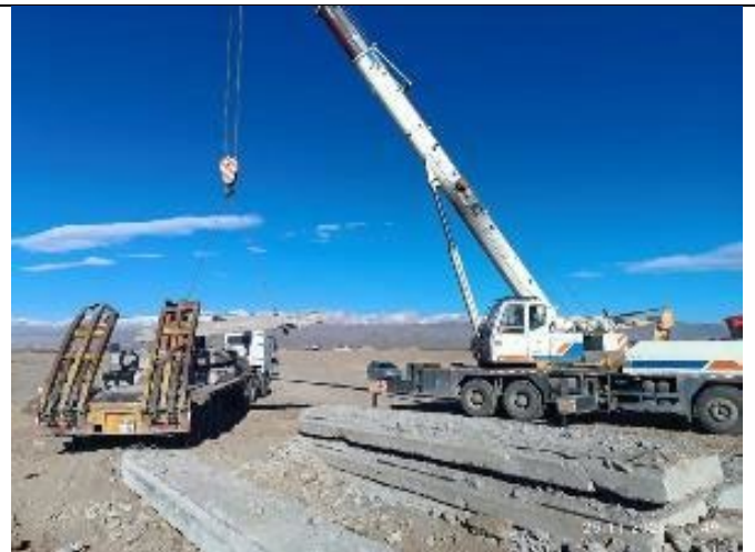
Photo 91. Removal of dismantled parts of temporary bridge for bypass road at km 62+500.
