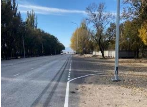
Photo 9. Lot 1, Laying of white edge marker line at km 0+060-3+000. October 2024.
