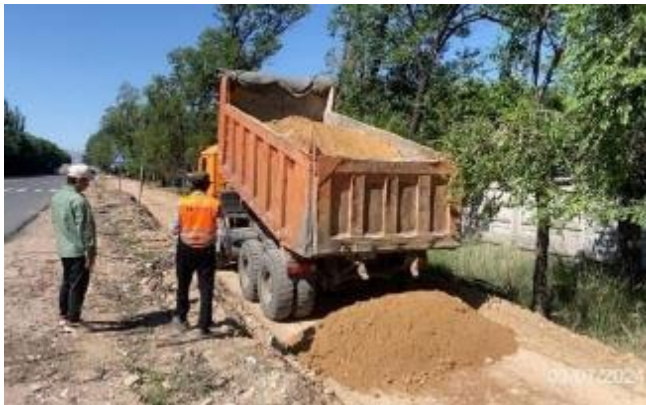
Photo 1. Lot 1. Embankment for sidewalk at km 1+950-2+100 RHS. July 2024.
